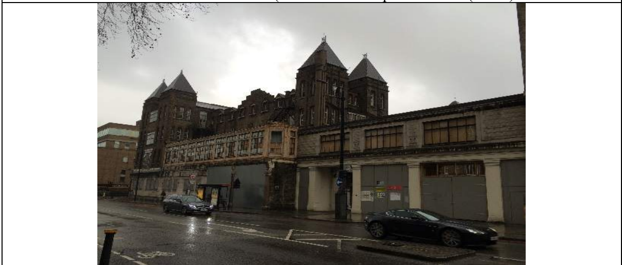
West Elevation of NTH
