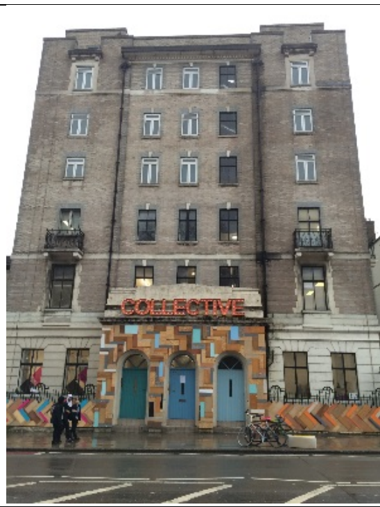
Insull Wing (Hampstead Road Elevation)
