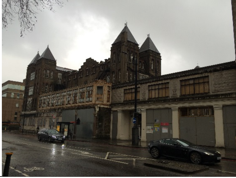
West Elevation (Vezev Wing)
