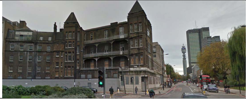
North Elevation (Vezev Wing) (view from Hampstead Road (A400))
