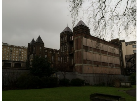
East Elevation (Vezev Wing)
