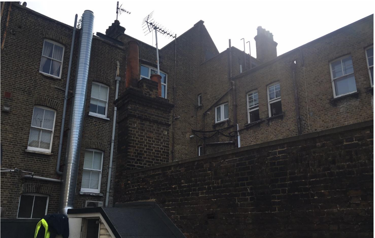
Figure 2; View of rear elevation including extract riser
