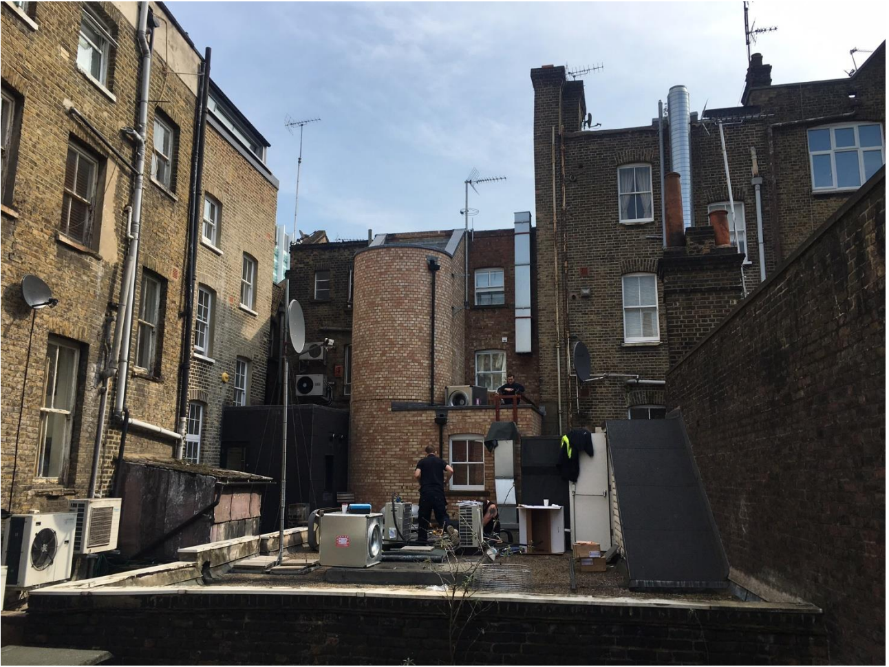
Figure 3; View of rear elevation incorporating plant equipment
