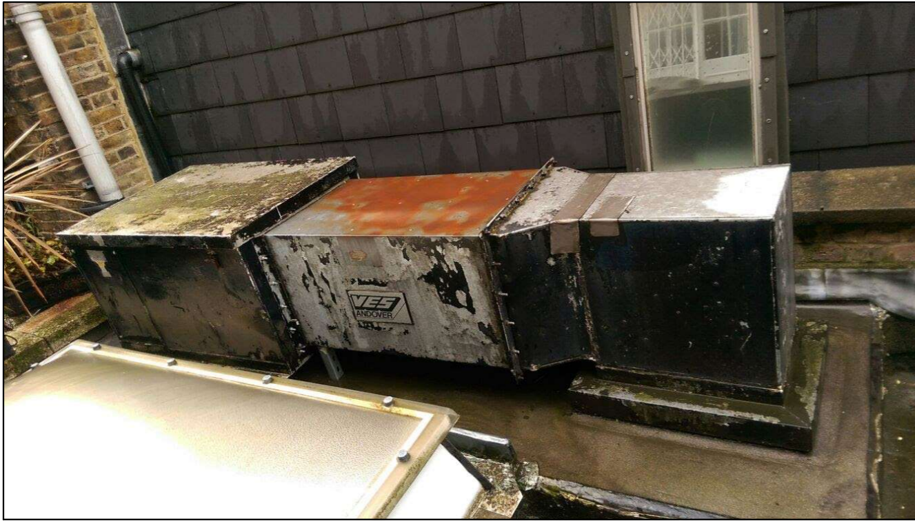
IMAGE 01- EXTRACTION UNIT AS PRE-EXISTED
