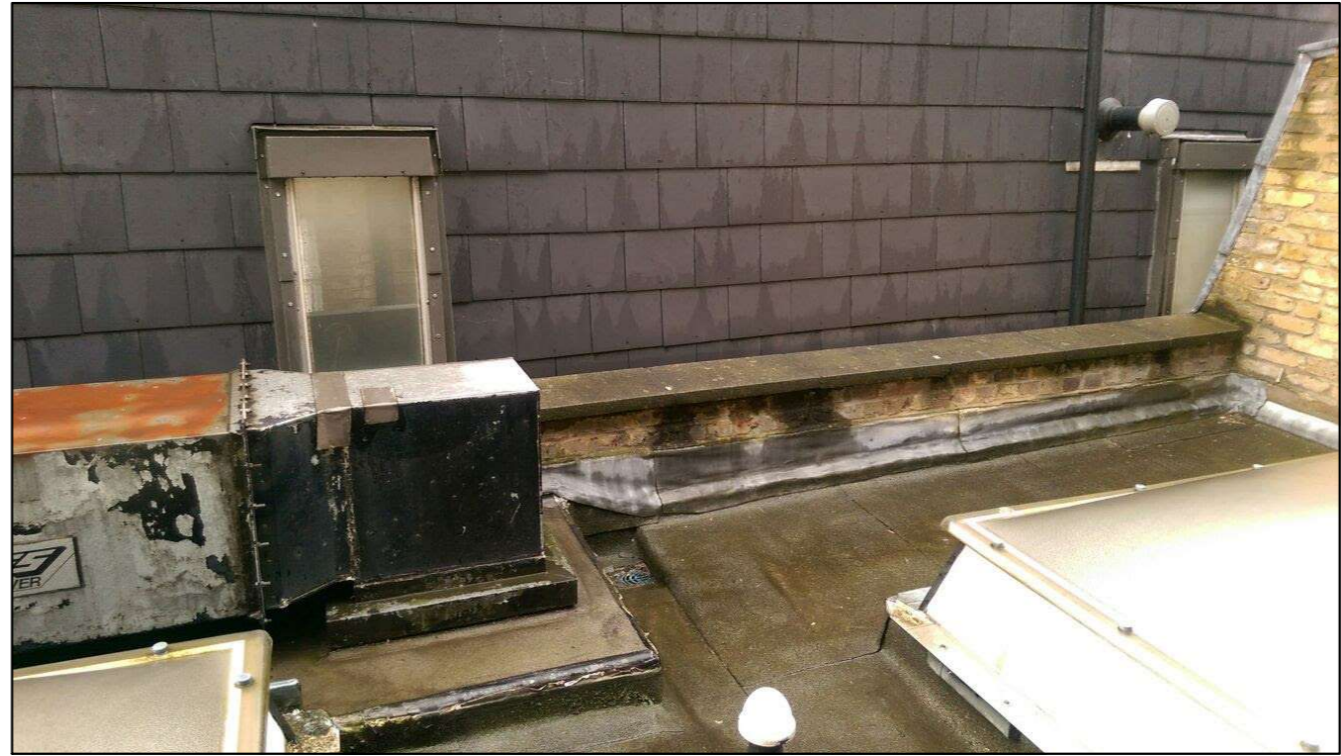
IMAGE 02- EXTRACTION UNIT AS PRE-EXISTED
