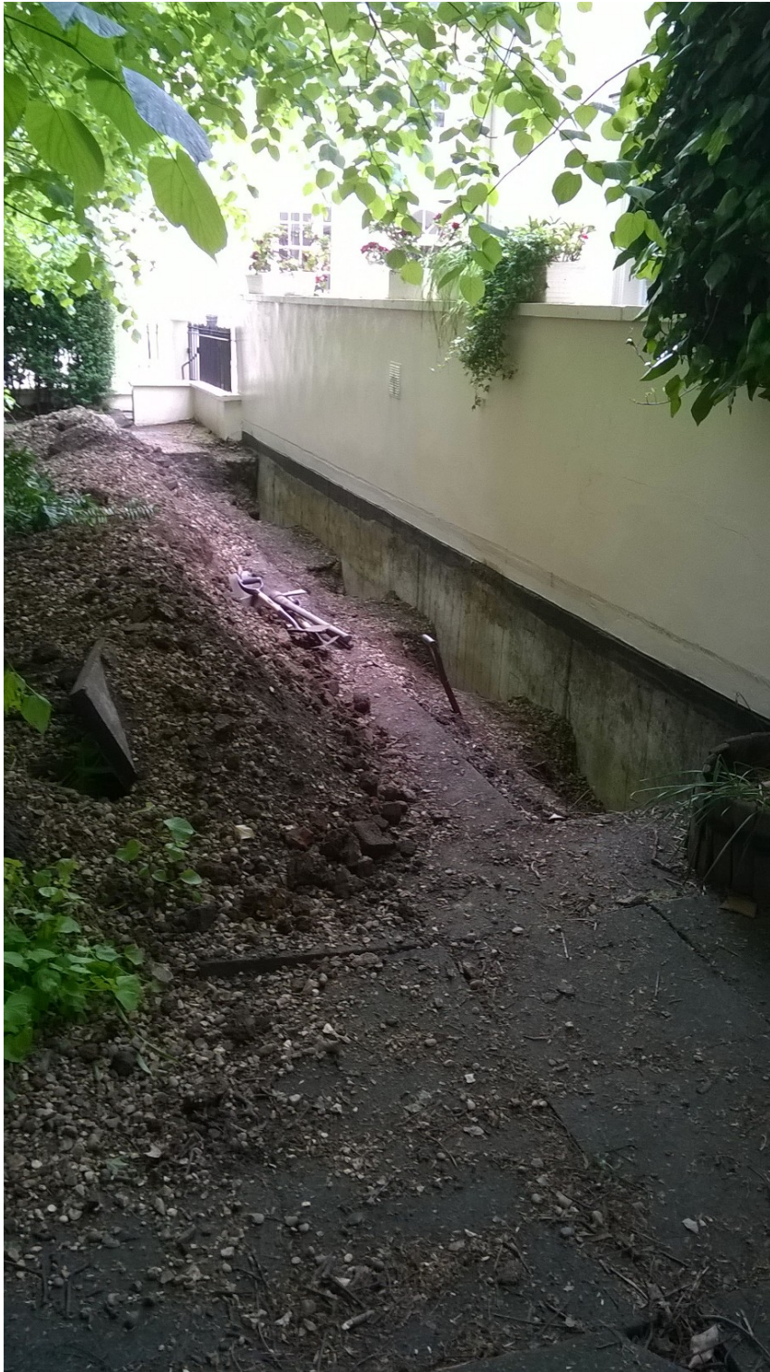
Photograph 4 – General view of trench alongside garage wall
