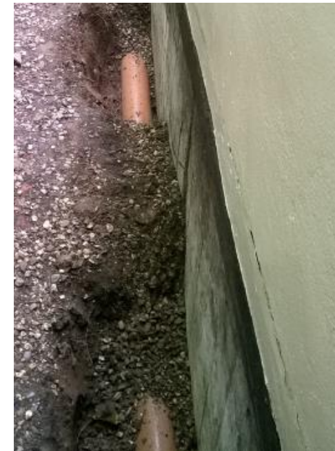
Trial trench photograph
