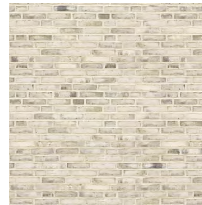
Light buff coloured brickwork with a whitewash creates a warm, soft varying surface texture
