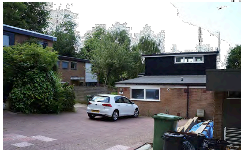
View of existing from entrance driveway adjacent to no.3
