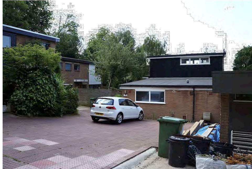
VIEW FROM UPPER LEVEL PARKING AREA
