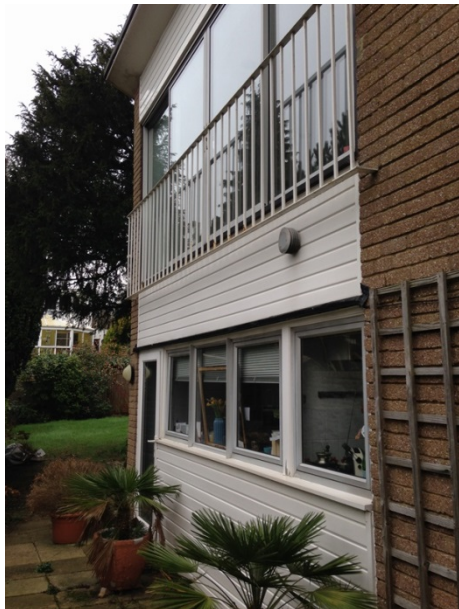
Rear view of property showing the lower ground floor at approximately garden level
