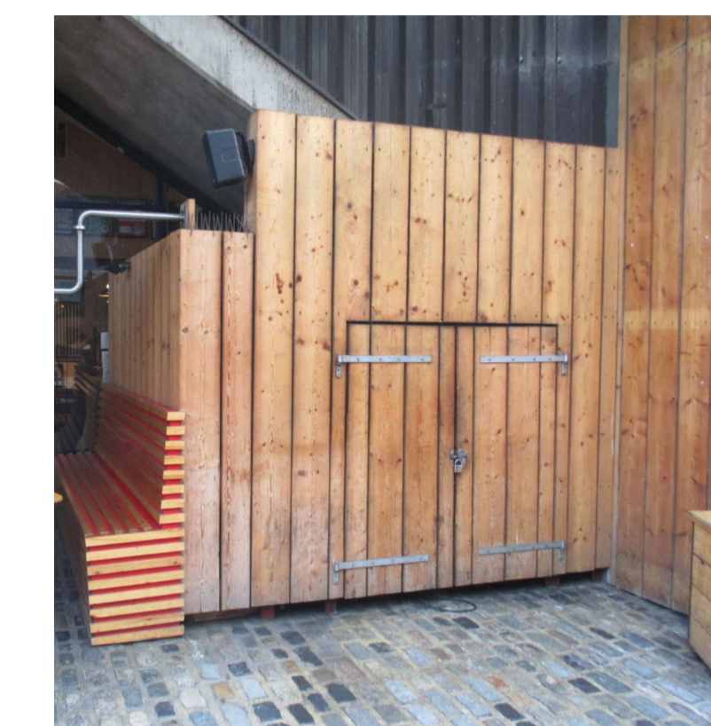
IMAGE OF EXISTING STORAGE UNIT
