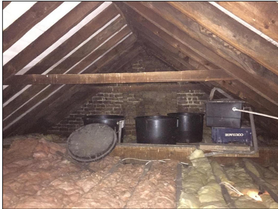
Photo App. 6.3 (above): Detail of the eastern (rear) roof looking towards the south of the building. Modern membrane visible over the timbers throughout with water storage tanks to the southern end.
