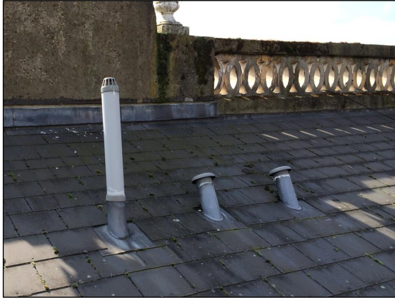
Photo App. 5.3 (above): Inside face of west façade of building roof area with likely non-original roof with 'modern' ventilation integral to the roof and the concrete inside facing/alterations to parapet.
