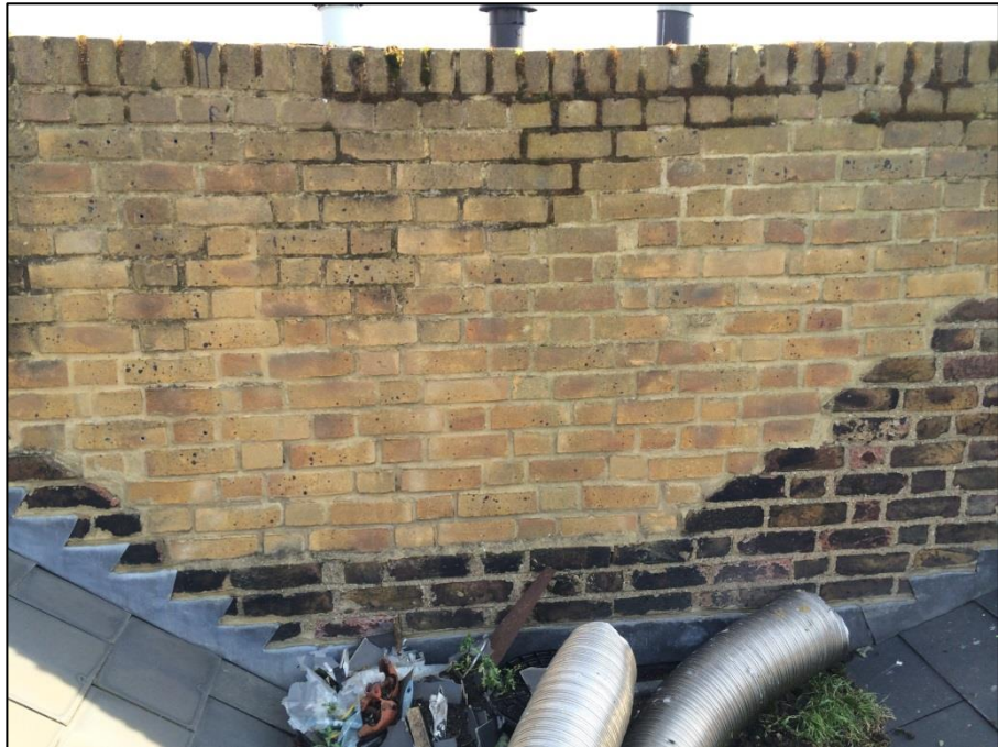
Photo App. 5.6 (above): Detail of the view towards inside face of south façade showing 'modern' new build-up of the party wall with the adjacent property.
