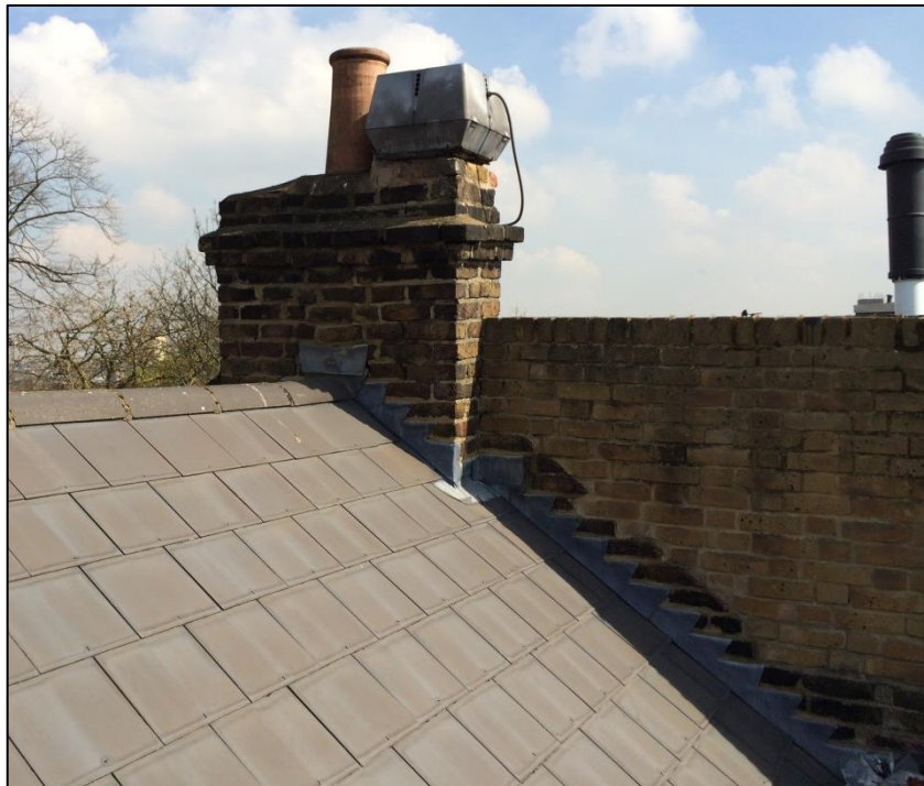
Photo App. 5.8 (above): Detail of the view towards inside face of south façade showing ‘modern’ new build-up of the party wall adjacent to the eastern (back) roof where the roof form/pitch may be original but all of the external roof fabric is later replacement likely from the mid to late 20 th Century.
