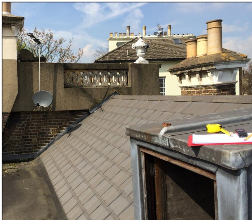
Photo App. 5.4 (above): Inside face of north façade and east portion of roof area with access hatch from roof space. Roof form may be 'original' but has been recovered with artificial slates and modern underlay. Also shows rendered facing/alterations to parapet.
