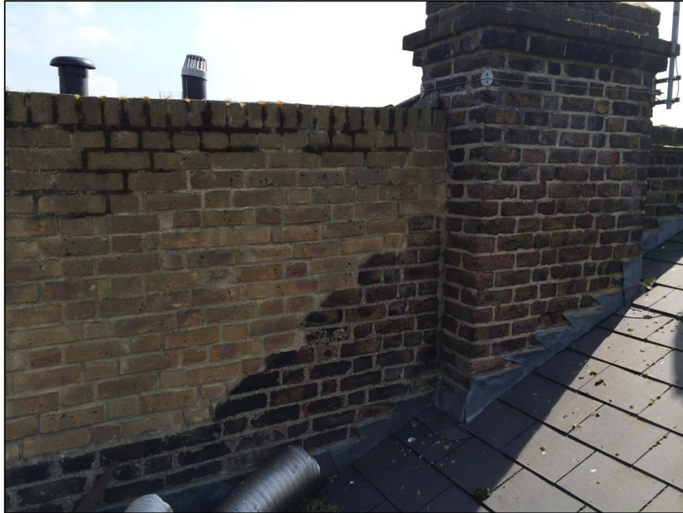
Photo App. 5.7 (above): Detail of the view towards inside face of south façade showing ‘modern’ new build-up of the party wall with the adjacent property and the cut bricks on a different angle to the current front roof suggesting an earlier roof has been replaced with the single slope of the front parapet.
