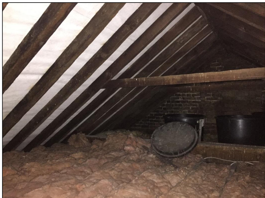
Photo App. 6.4 (above): Detail of the interior of the eastern (rear) roof looking towards the south of the building. Modern membrane visible over the timbers throughout.
