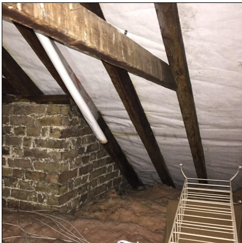
Photo App. 6.6 (above): Interior of eastern (rear) roof at junction of part of the rear wall where the roof extends further to the rear with modern waterproof membrane over the timbers of the roof. Confirming much of the 'exterior' fabric is late 20 th Century alteration/roof replacement.
