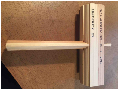
PROPOSED REPLACEMENT SASH MOULDING (STRETCHED OVULO)
