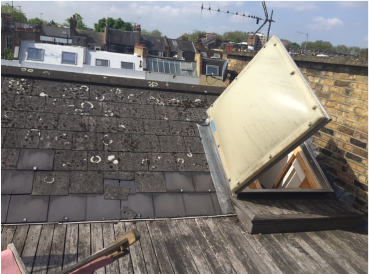
Photo 2 – View of the area to be extended
