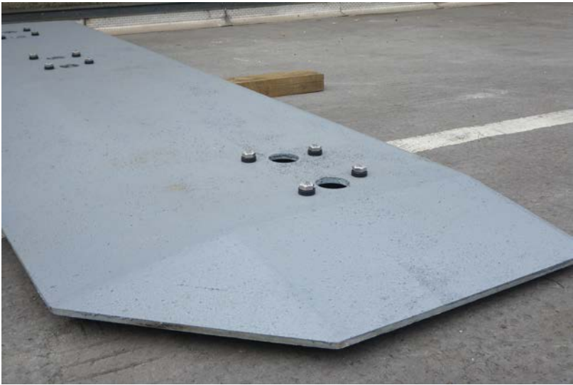
Figure 2.5: Prototype of surface mounted platform (ramped end) showing fixing bolts for street furniture. Ramp is artificially raised for visibility. The platform shows the correct colour, but a different paint system.
