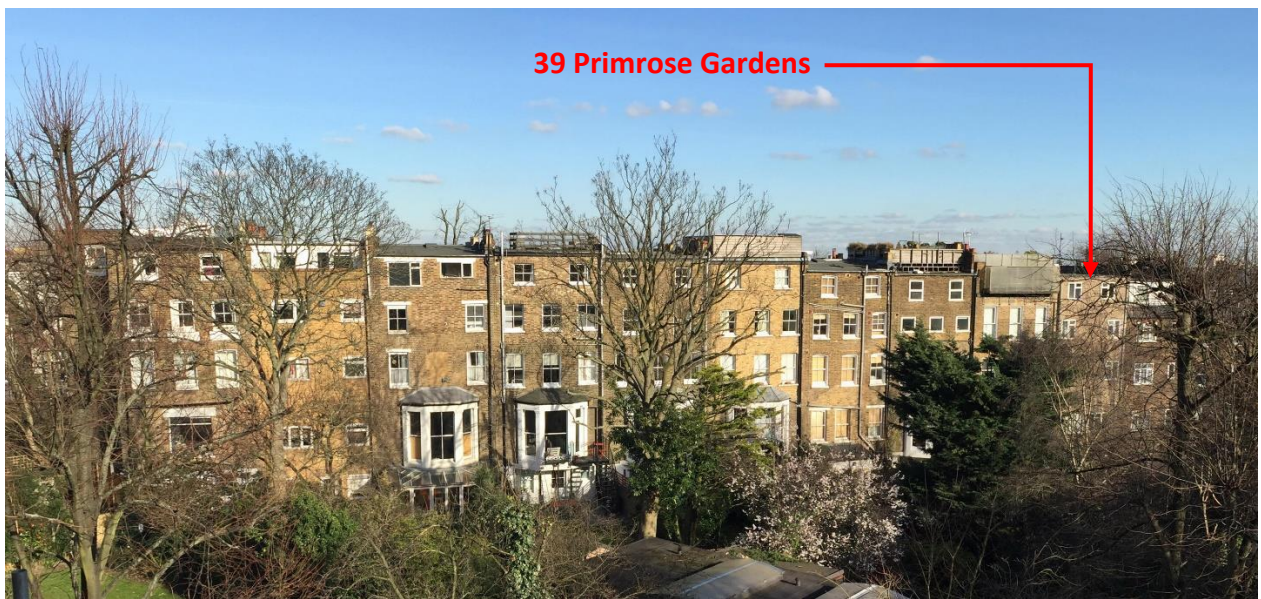
Rear view of Primrose Gardens from 6 Belsize Grove
