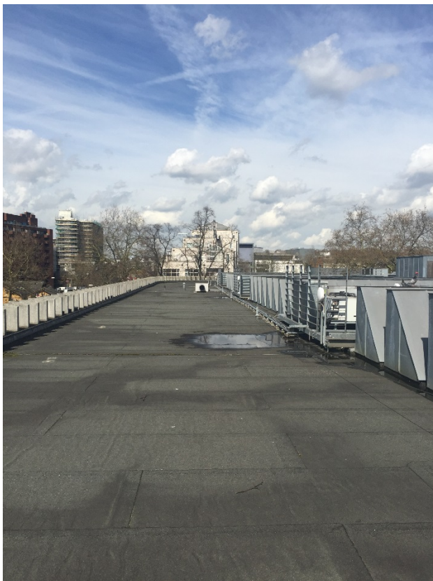
Figure 6: Asphalt Roof and Surrounding Parapet
