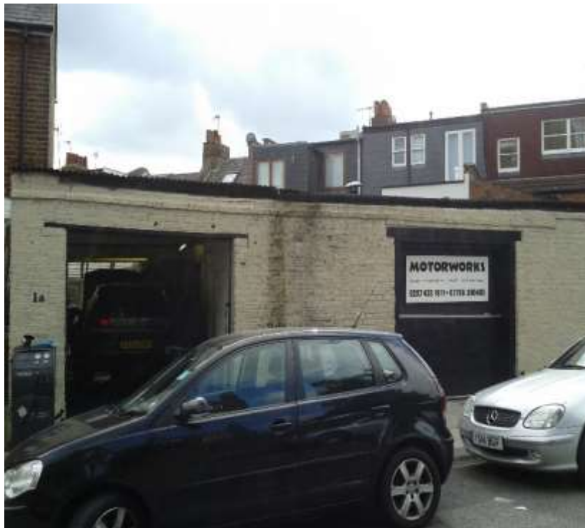
Figure 2 – Existing building on development site
