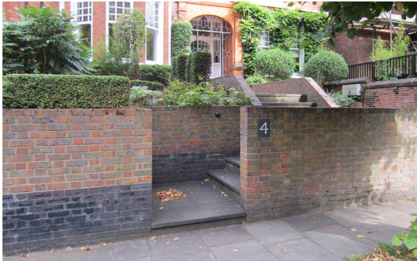
14 4 Wedderburn Road Pedestrian Entrance
