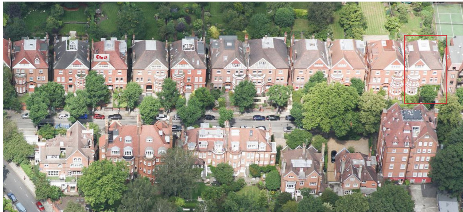
1 Aerial view of front of no.4 Wedderburn Road
