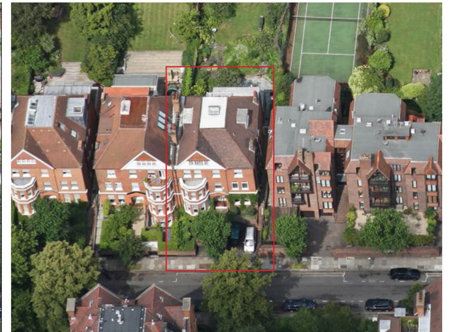
2 Aerial view of front of no.4 Wedderburn Road
