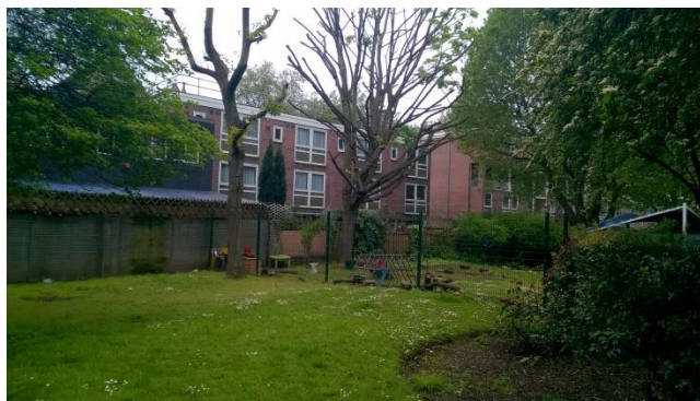
Figure 4: Rear of Laxton Place Properties
