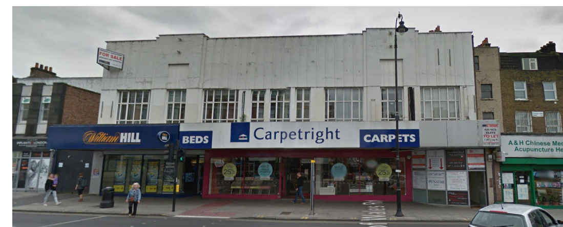
Photo of West Elevation
