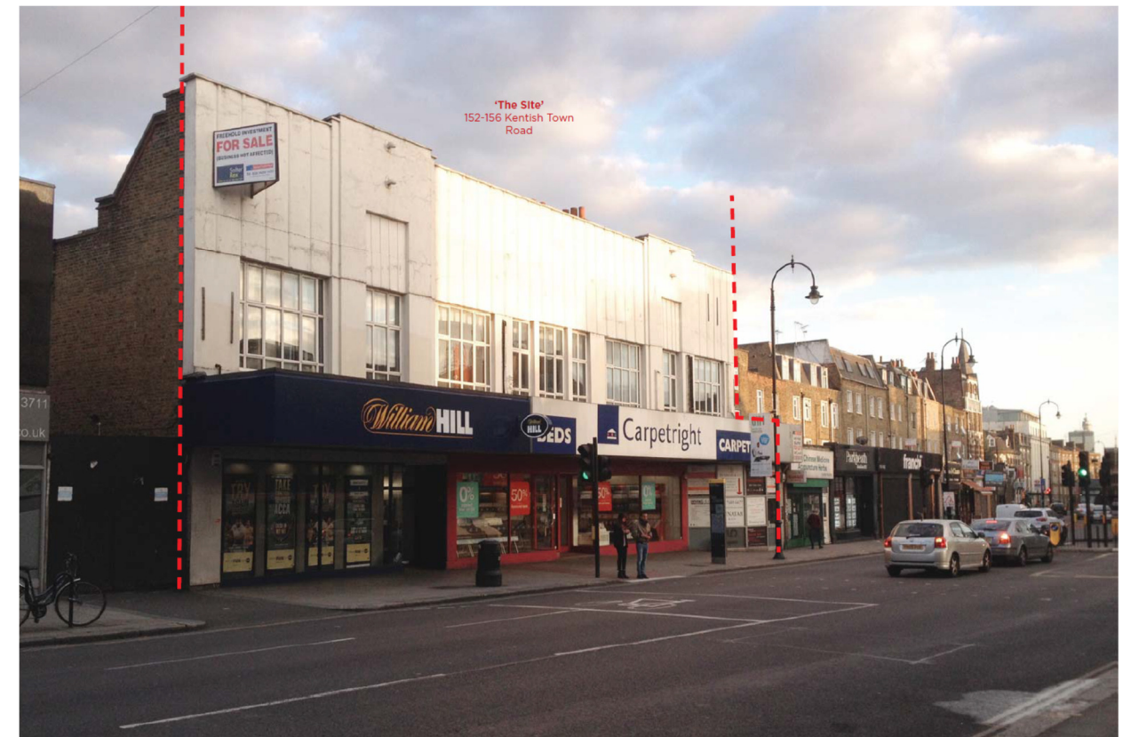
Street level view of West façade from North West
