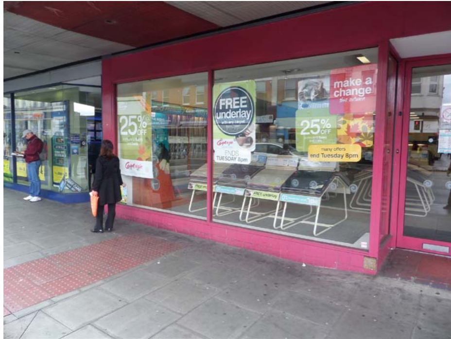
1. 152-156 Kentish Town Road Existing shop fronts
