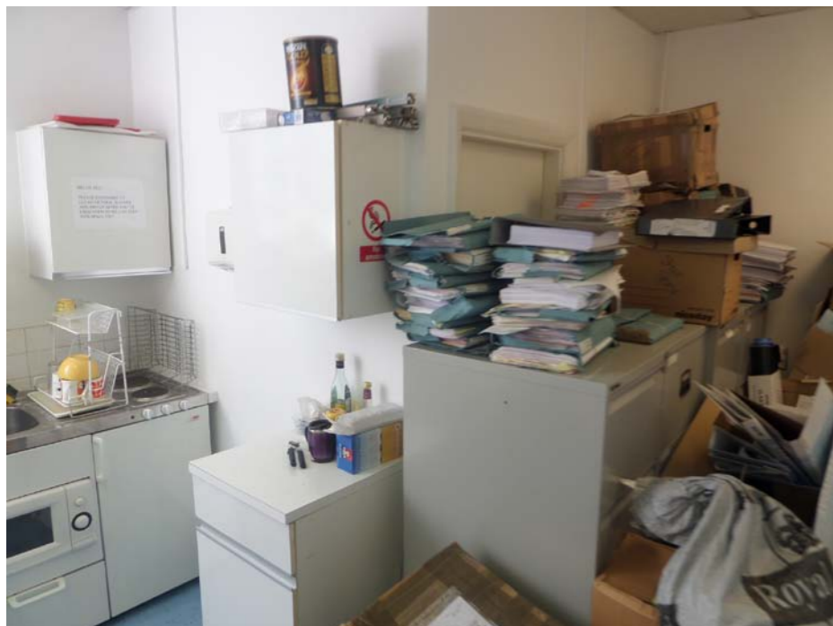
3. 152-156 Kentish Town Road Existing first floor office's kitchenette
