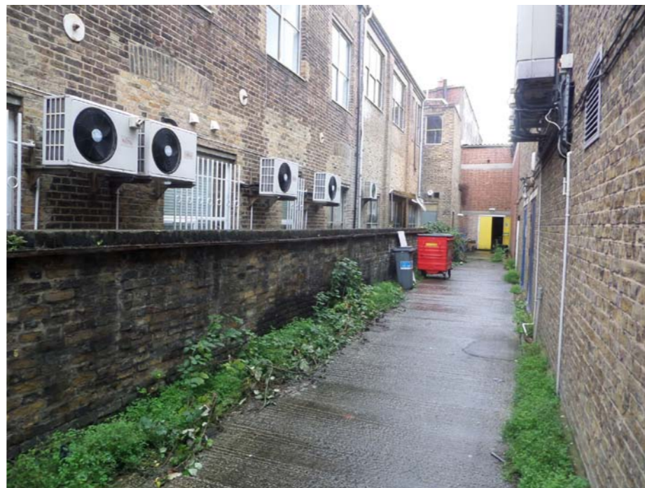
3. 152-156 Kentish Town Road Service Road
