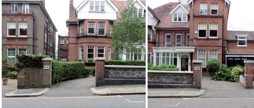
Figure 1: Double 'in and out' gateways are a typical historic feature (originally to allow horse drawn carriages to enter and leave properties).
