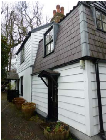
Image 20 - Existing rear canopy
