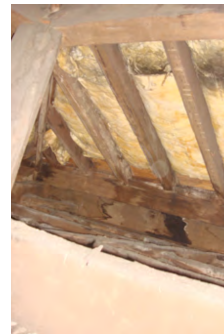
Figure 133 (above): King Post Truss above Room 206, No. 2 Roof. Figure 135 (below): Purlin, rafters, wall-head plate from south side above Room 206, No. 2 Roof. .
