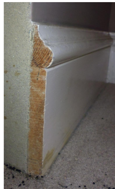
Existing skirting from room 3.03
