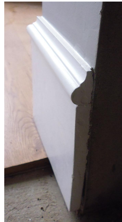
Existing skirting from room 2.03
