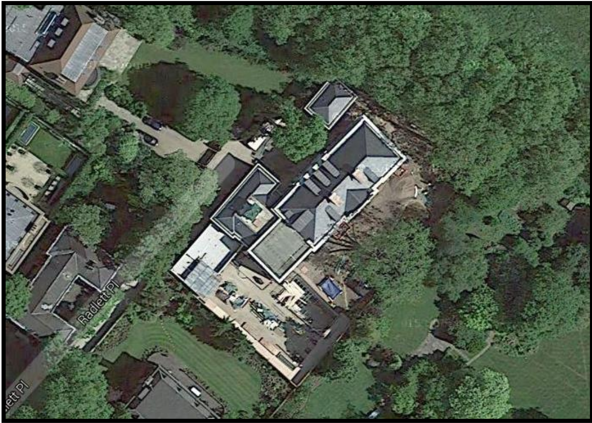
Figure 2: Aerial image of site
