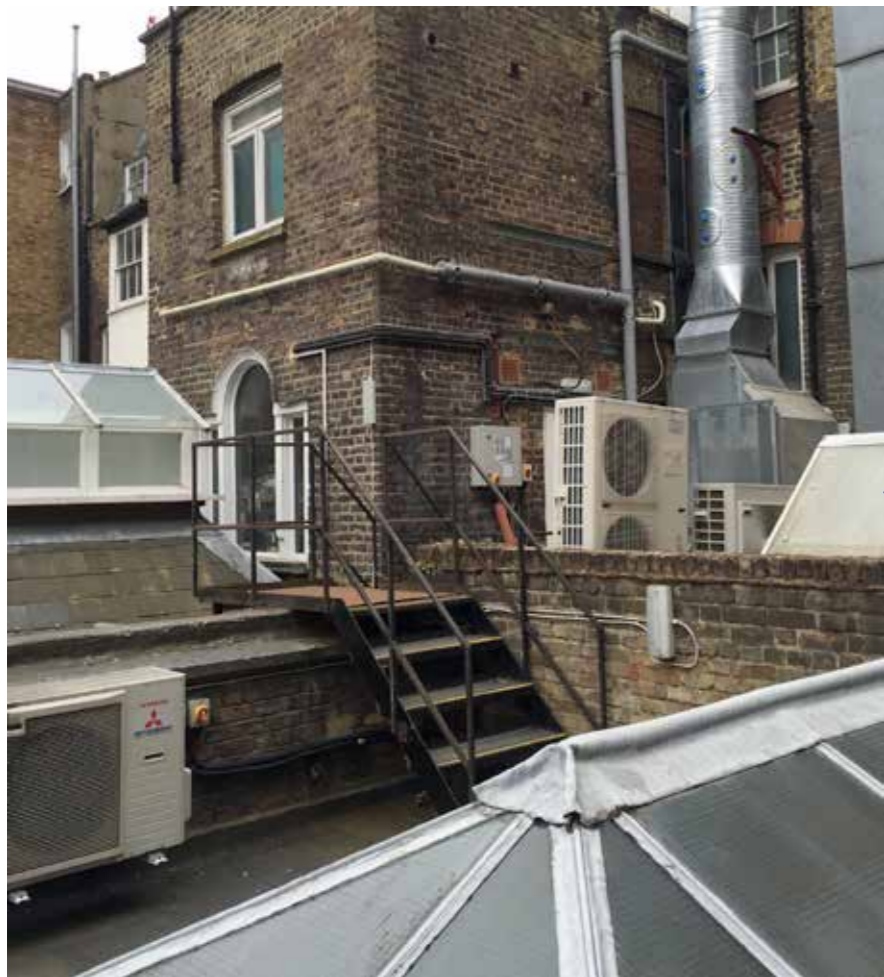
FIRE ESCAPE STAIRS
