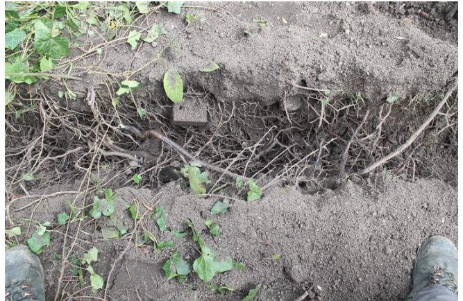
Photo 58. Trench 5 Section B.
