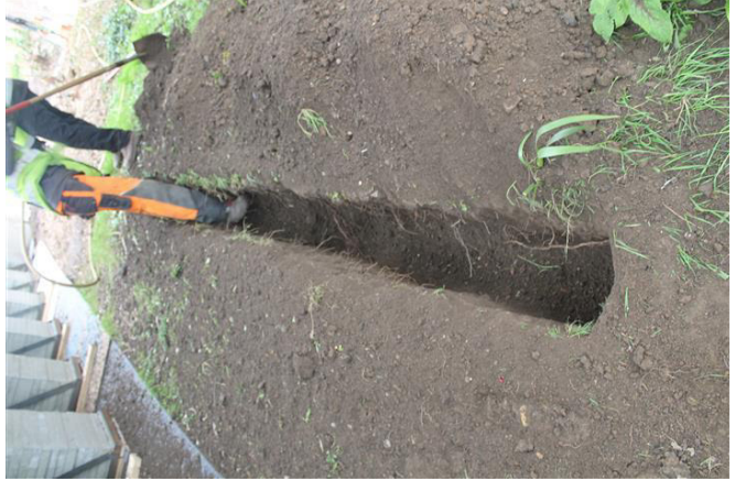
Photo 74. Start of excavation for Trench 7.
