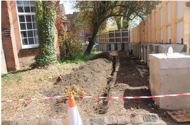
Photo 75. Overview of Trench 7.
