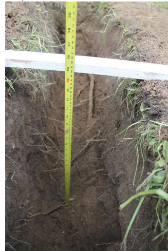
Photo 64. Depth of Trench 6 at 600mm.
