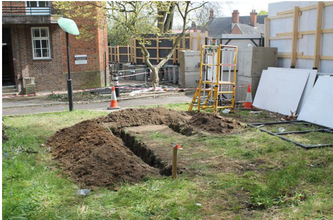
Photo 63. Overview of trench 6.
