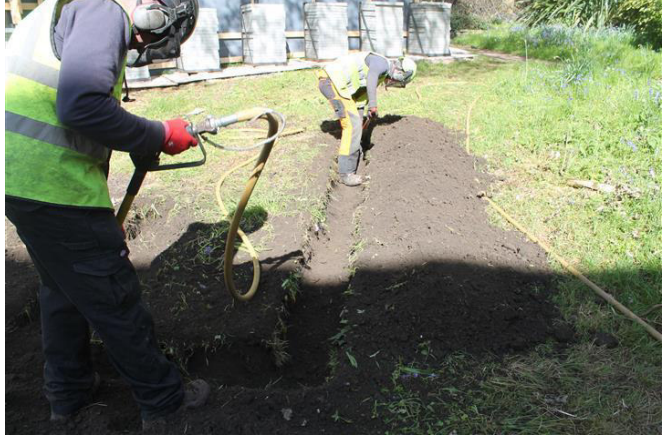
Photo 62. Start of excavation for Trench 6.
