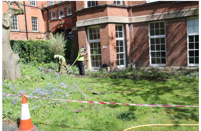
Photo 30. Start of excavation for Trench 3.
