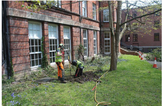
Photo 40. Start of excavation for Trench 4.
