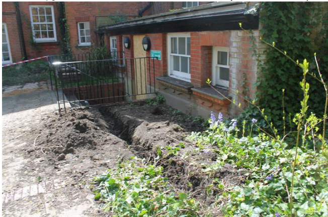
Photo 53. Start of excavation for Trench 5 (Sections A & B).
