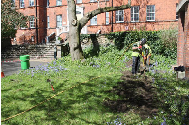
Photo 31. Overview of Trench 3.
