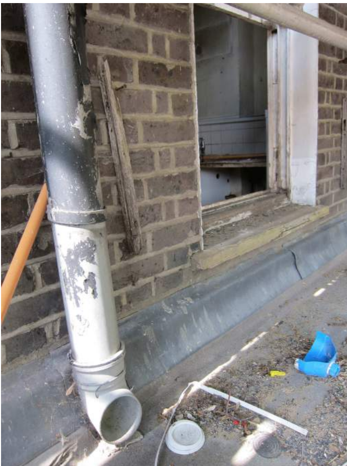
Rear elevation detail – plastic RWP discharges on to projecting shop roof, with window to first floor kitchen behind
