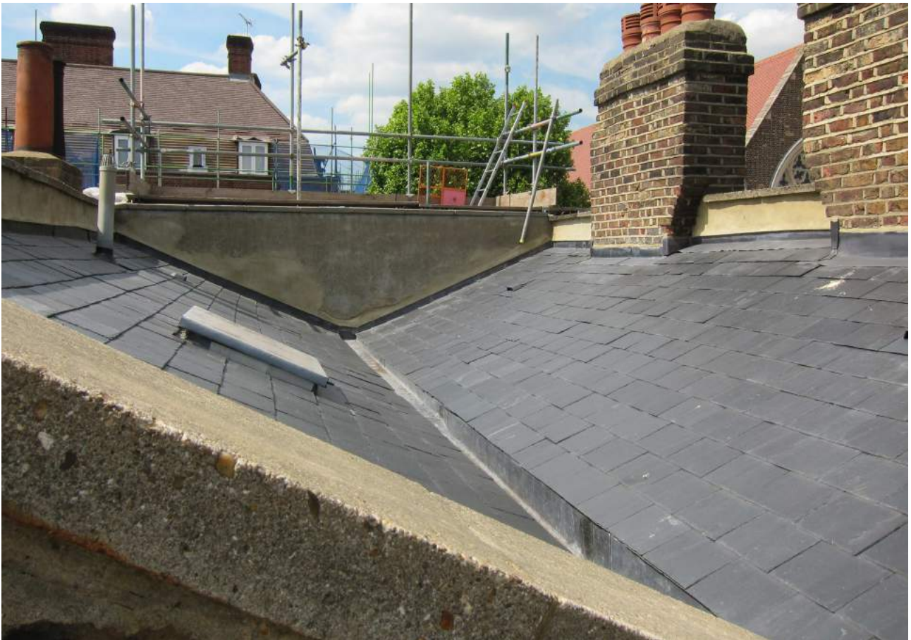
Roof, with replacement roof slates and lead-lined valley gutter
