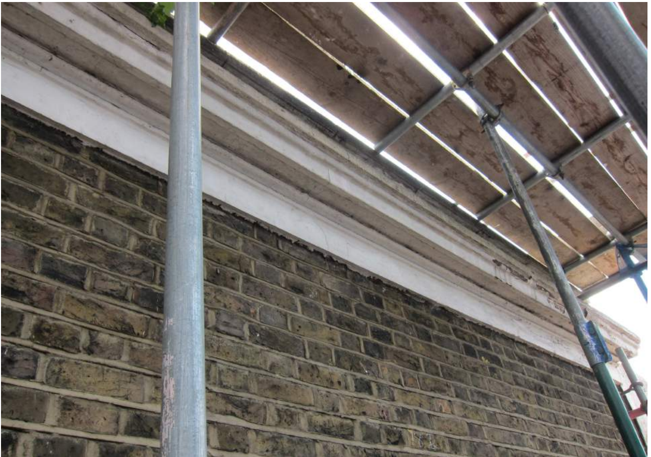
Stucco cornice to street elevation parapet
