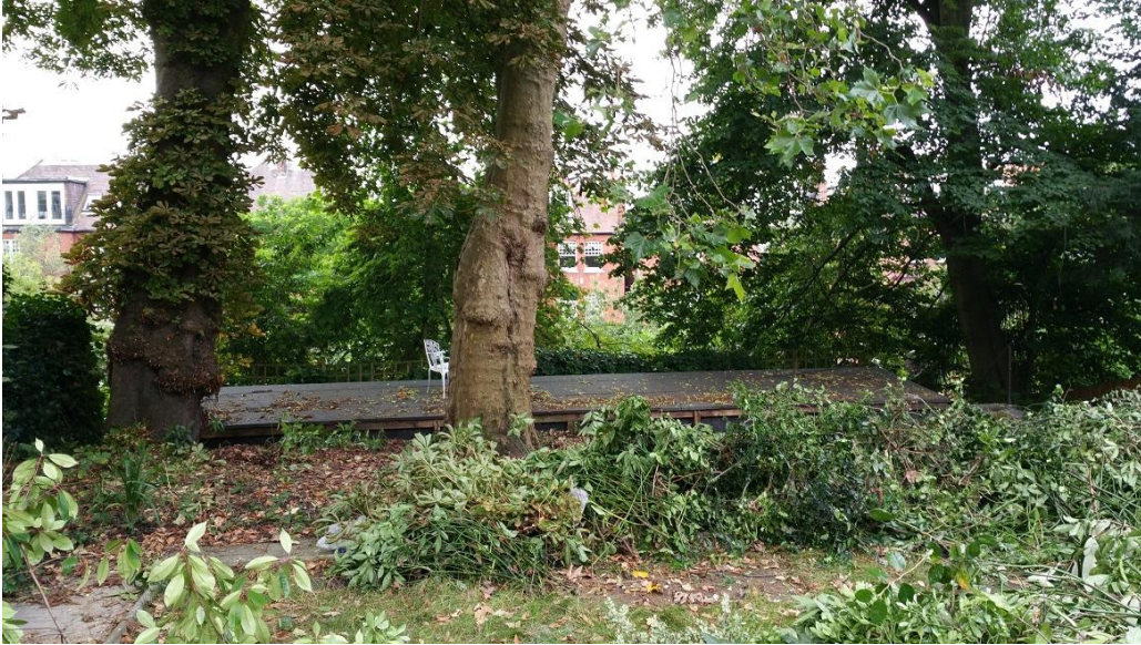
Photo 1 – Garden terrace area prior to installation of timber deck and glass balustrade.
