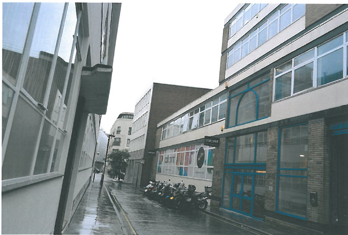
Plate 1 – Application building looking north
