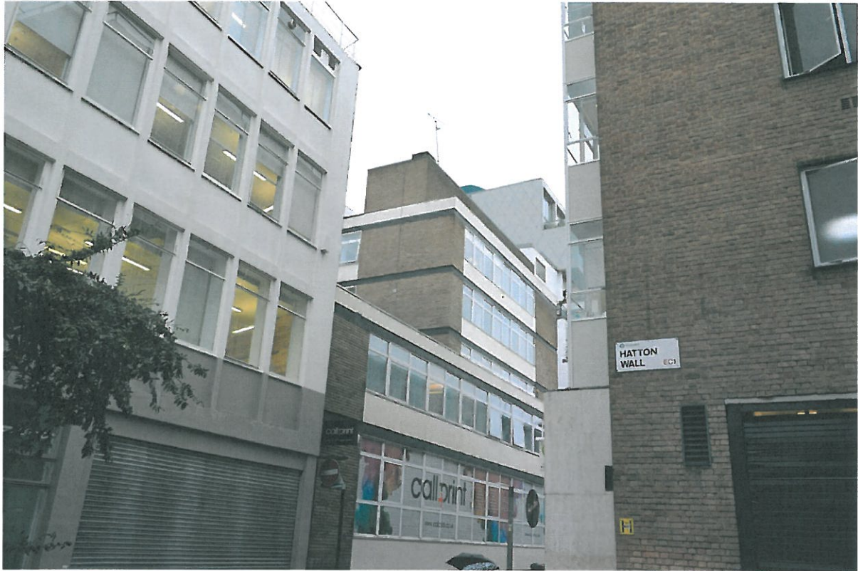
Plate 2 – Application building looking south
