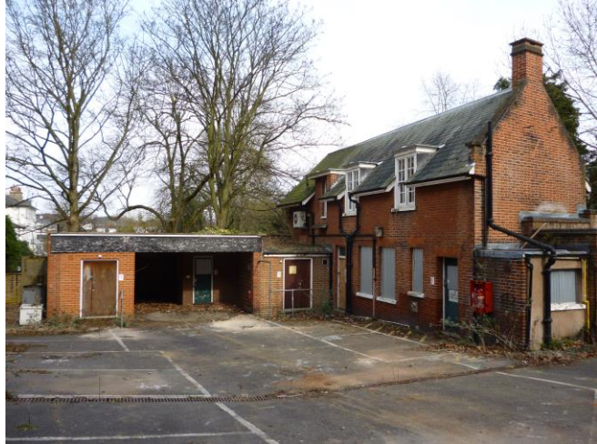
Photograph 1 Building 1, west and northern elevations.
