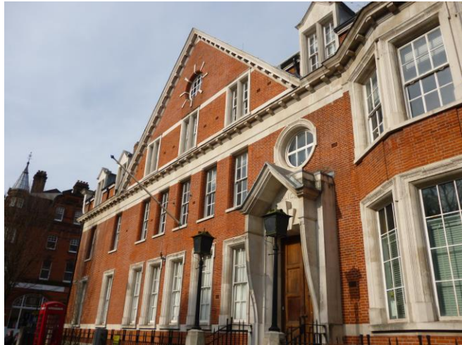
Photograph 2 Building 2, western elevation.
