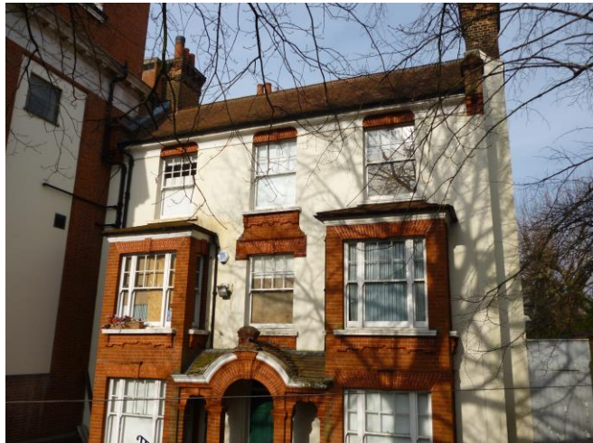
Photograph 3 Building 3, western elevation.
