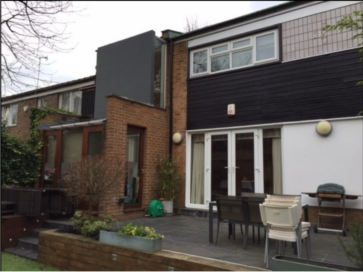
REAR SIDE GARAGE EXTENTION EXISTING LOOKING L
