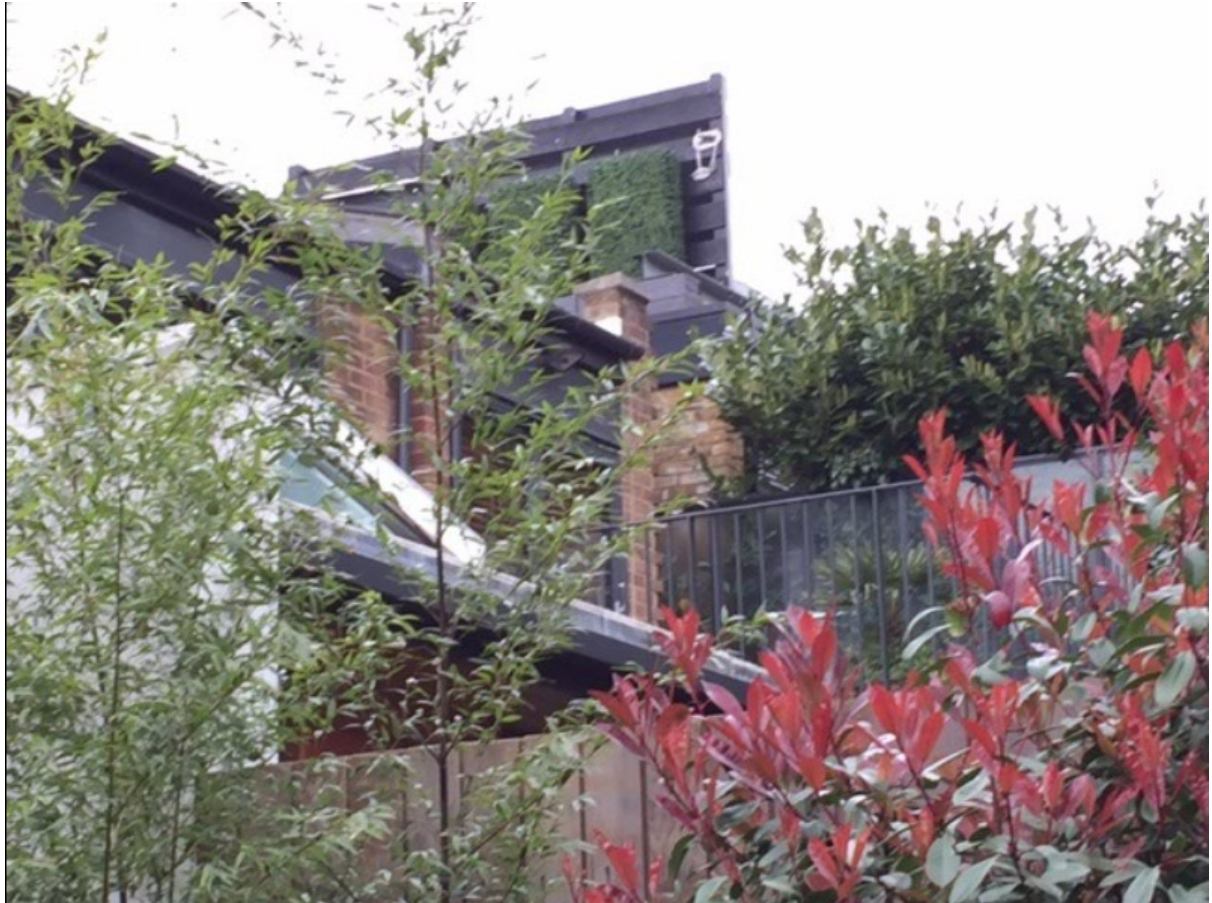
VIEW OF ROOF TERRACE AND SCREENING OF NUMBER 47 FROM NO 43 REAR
