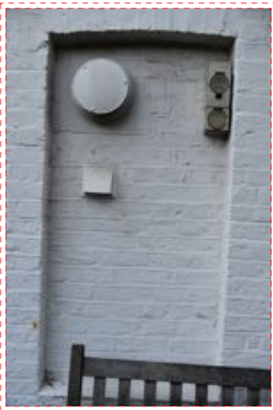
LGF utility room covered window.
