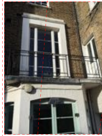
LGF extension balcony, seen from rear garden.
