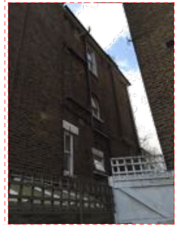
Facing north east, security gate detail.
