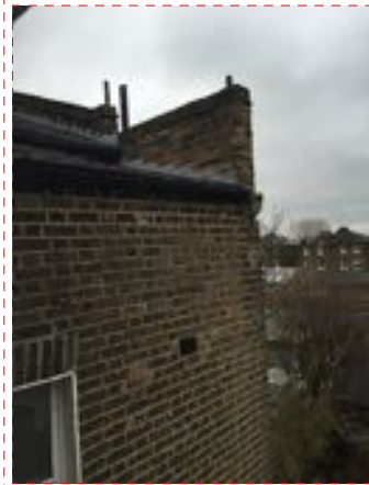
Second floor facing east roof detail.
