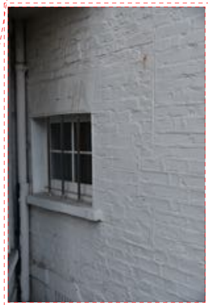
LGF utility room window.
