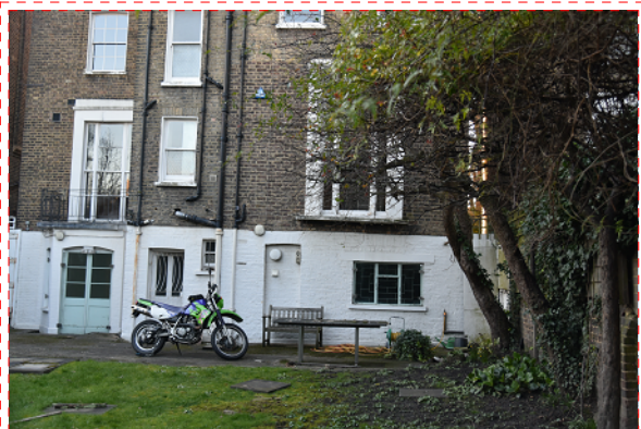
North lower facade (right hand side), kitchen window to the right.
