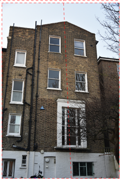
North facade (right hand side).
