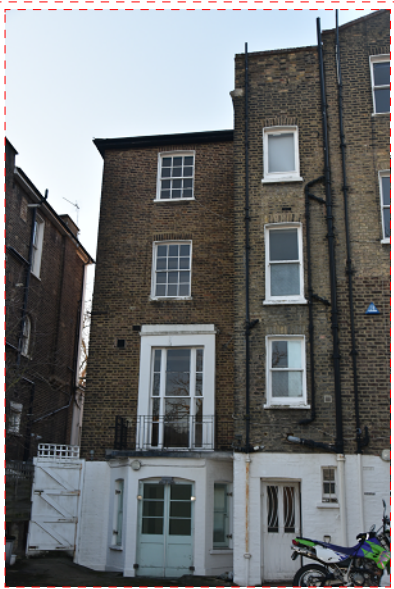
North west facade (left hand side).
