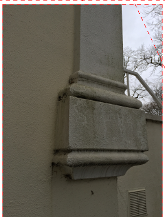
Front door extension left hand side ornamental pilaster base.
