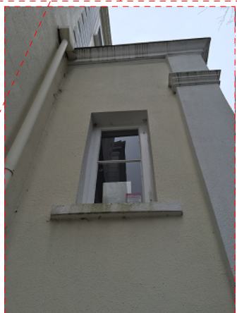
Front door extension left hand side window. Similar on the other side.
