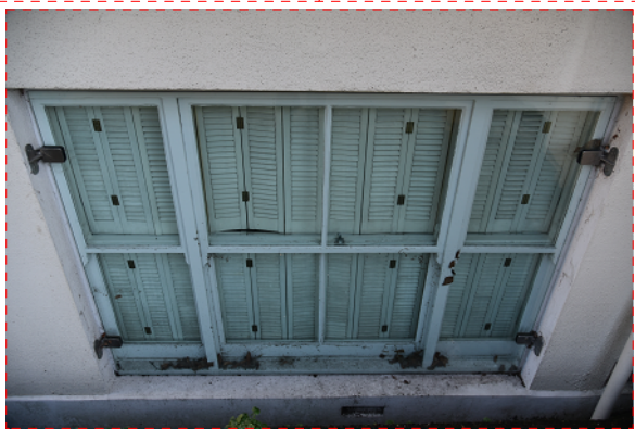
Front elevation left hand side window. Covered in security glass with temporary fittings.
