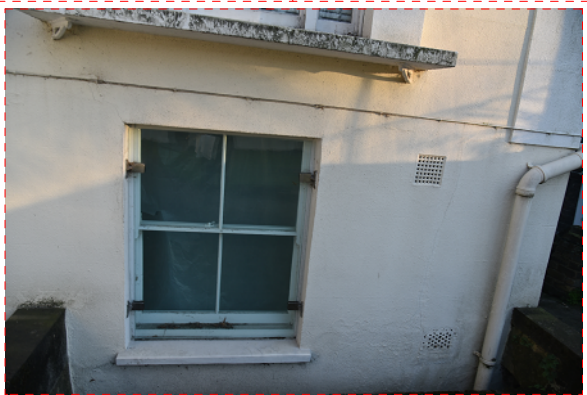
Front elevation right hand side window. Covered in security glass with temporary fittings.
