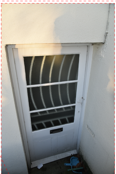
Front elevation right hand side lightwell door to LGF.
