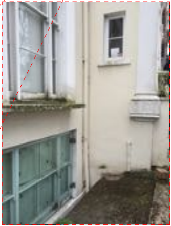
Facing south, left hand side of front door extension.
