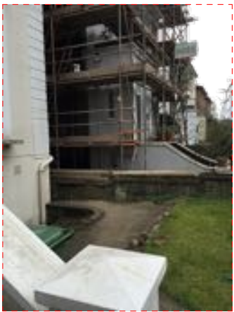
Looking South at concrete in front garden adjacent to house.
