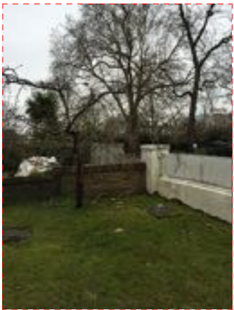
North west front garden, garden wall meets front wall.
