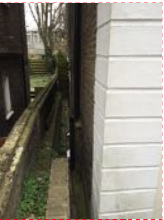
Facing south east, windows only on LGF.
