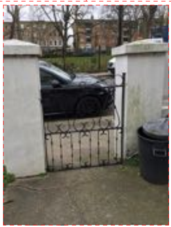
Front garden gate, facing Camden Square.
