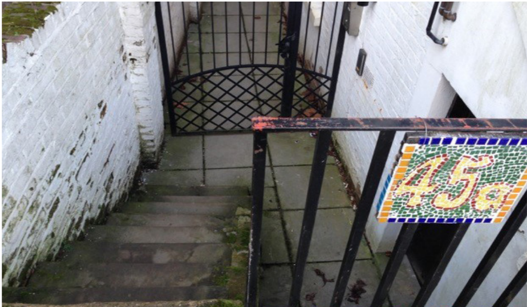
Steps to basement entrance
