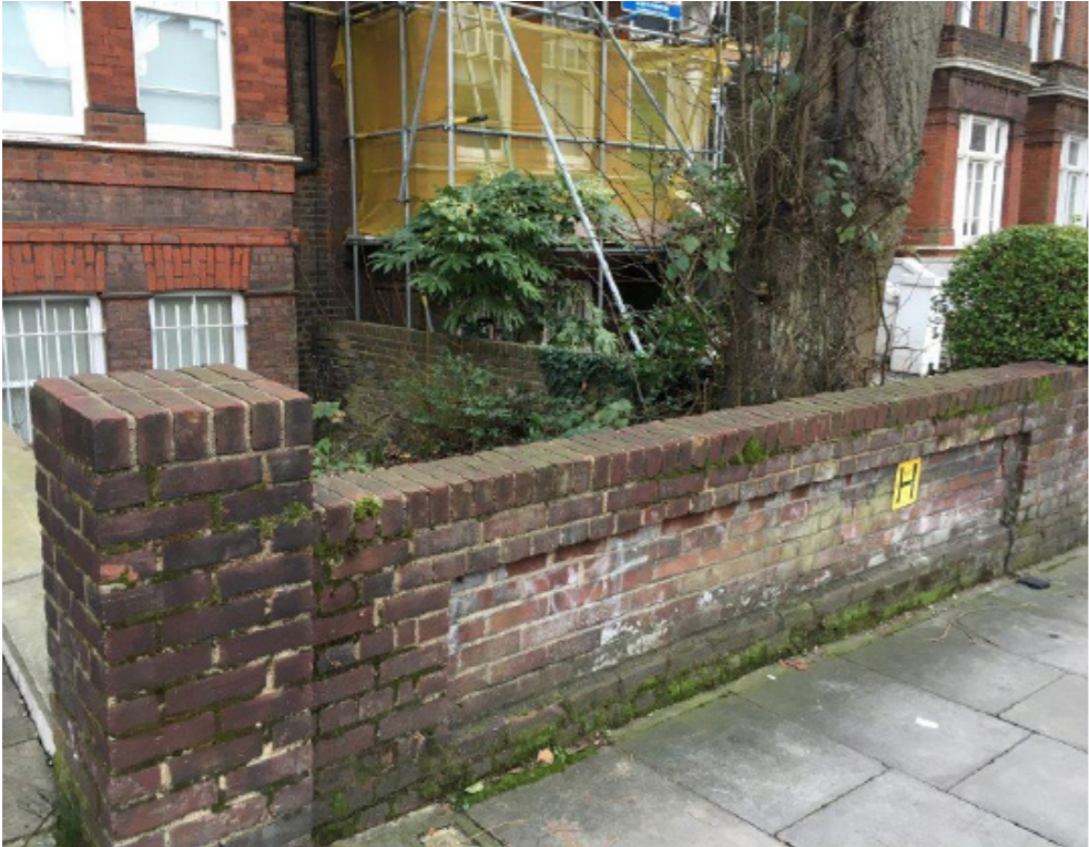
Street garden wall
