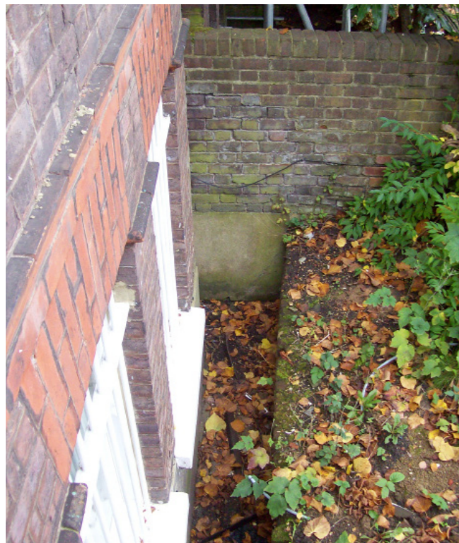
Basement well in front of windows
