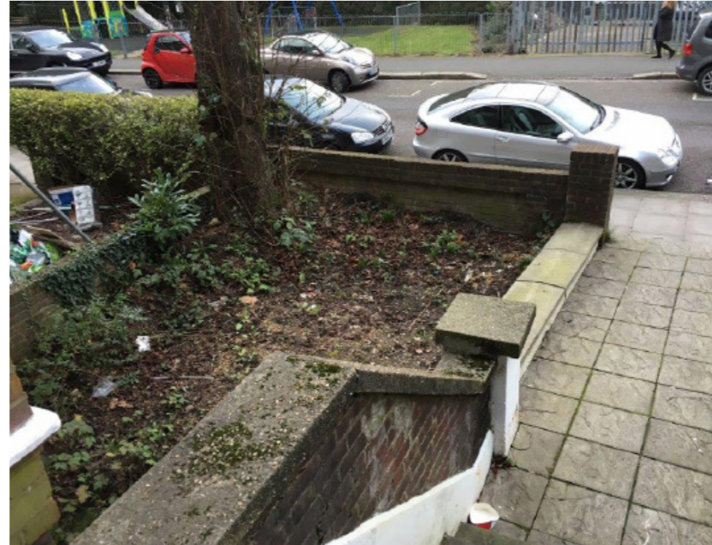
Looking from the front door
