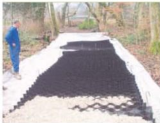
CellWeb during installation.
