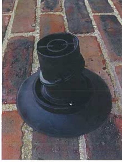
PHOTO 9 – Boiler outlet To side wall – recessed position
