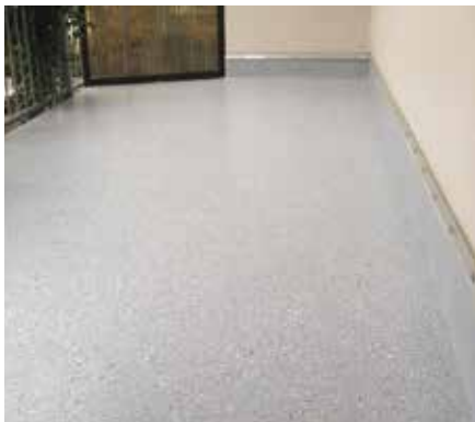
Below: New light grey balconies
