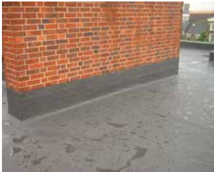
Above: Dark grey roof refurbishment
