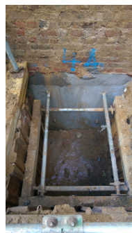
1 SOUTHWICH YARD, W2, UNDERPINNING/ RETAINING WALLS New residential Lower Ground floor
