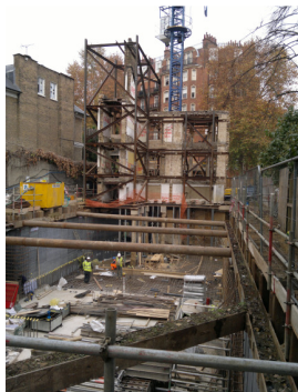
60 Addison Road W14, Facade retention over new basement
