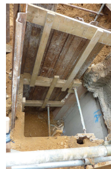
1 SOUTHWICH YARD, W2, UNDERPINNING/ RETAINING WALLS New residential Lower Ground floor
