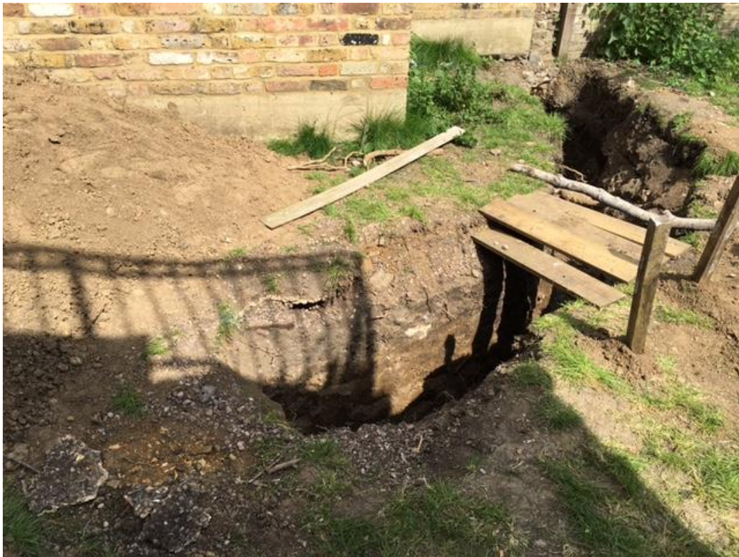
Fig.2 View of excavated trench
