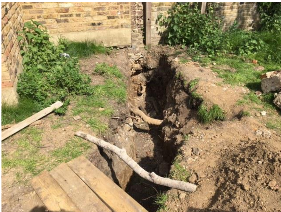
Fig.3 View of trench showing single large root at approx. 90cms depth
