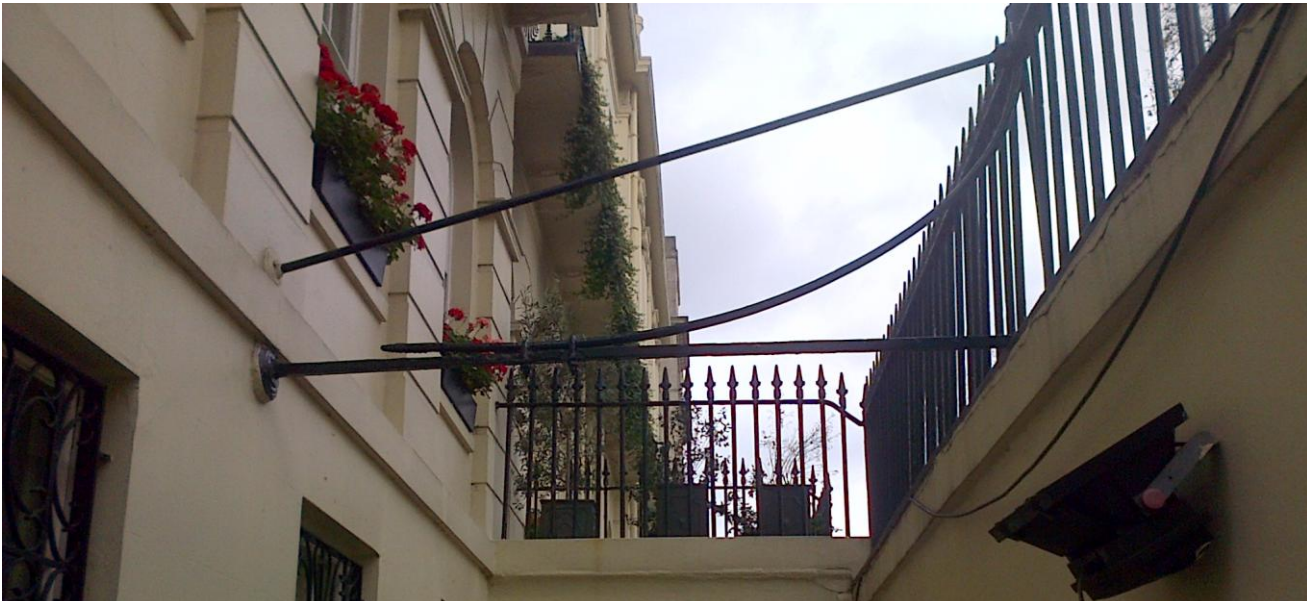
Photo 14: Step access to lower ground floor outside space.
