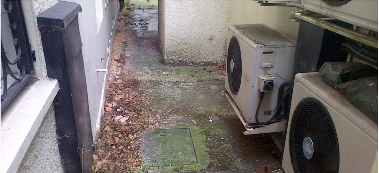
Photo 10: Lower ground floor outside storage space.
