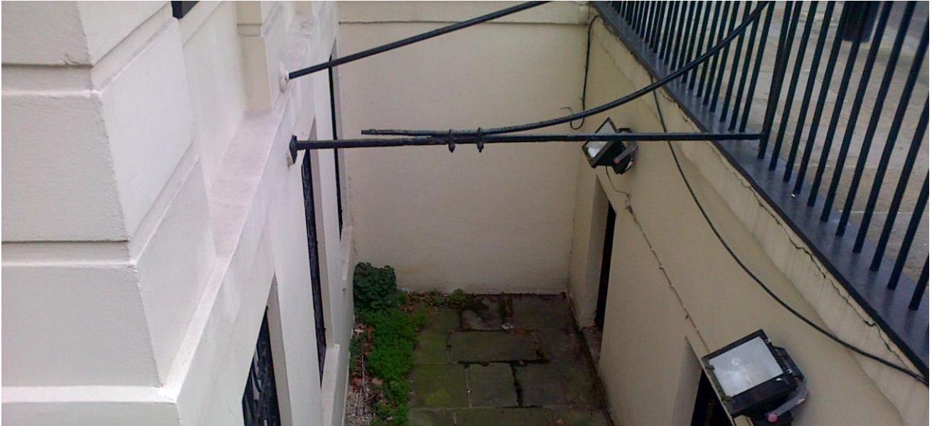
Photo 16: Patio area as viewed from ground level.
