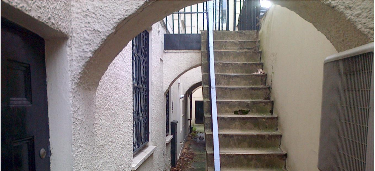
Photo 8: Access to from side of property to rear patio (width restriction).
